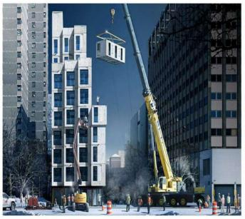
Like Tokyo, in Manhattan space is at a premium. My Micro NY is the city's first micro-apartment building and, consisting completely of modular units, was one of the first multi-unit Manhattan buildings to use off-site construction. At nine stories tall and 35,000 square feet total space, the building features 55 modular units
